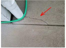
Acceptable Acceptable Needs Repair Steps/Stoops: Concrete Porch: Concrete Patio: Concrete - Crack in concrete, recommend filling to avoid further damage, Heavily cracked and unevenly settled causing trip hazard
